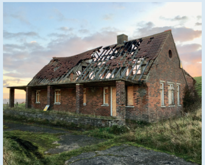
ROTOR bungalow on the Goldsborough road
